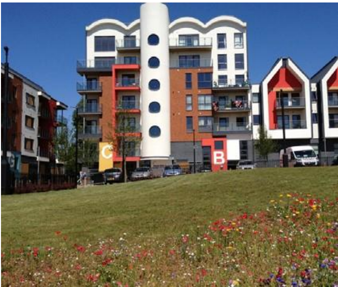
Architecture and green space works together to generate character in Bristol
